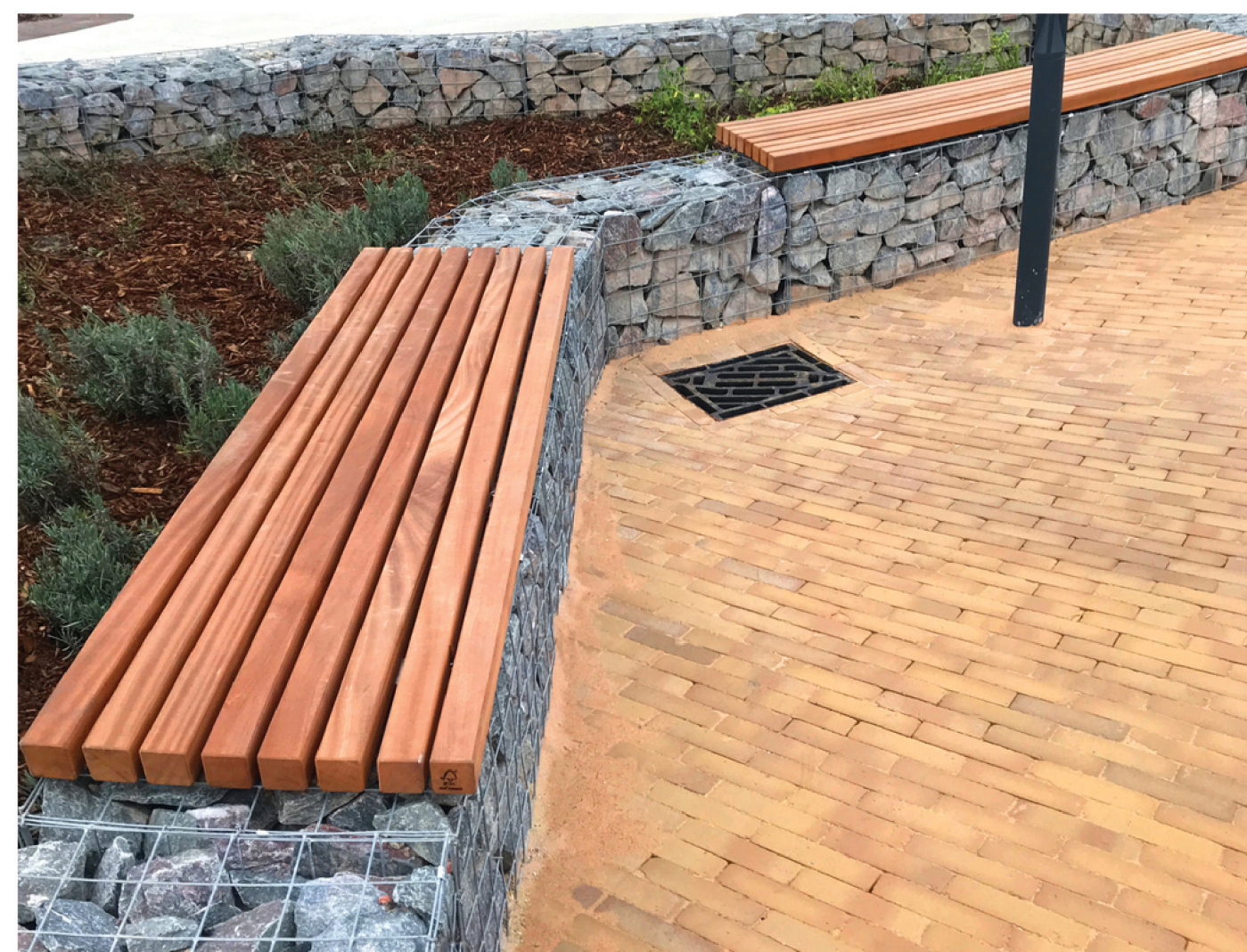
Gabion Seat Walls
